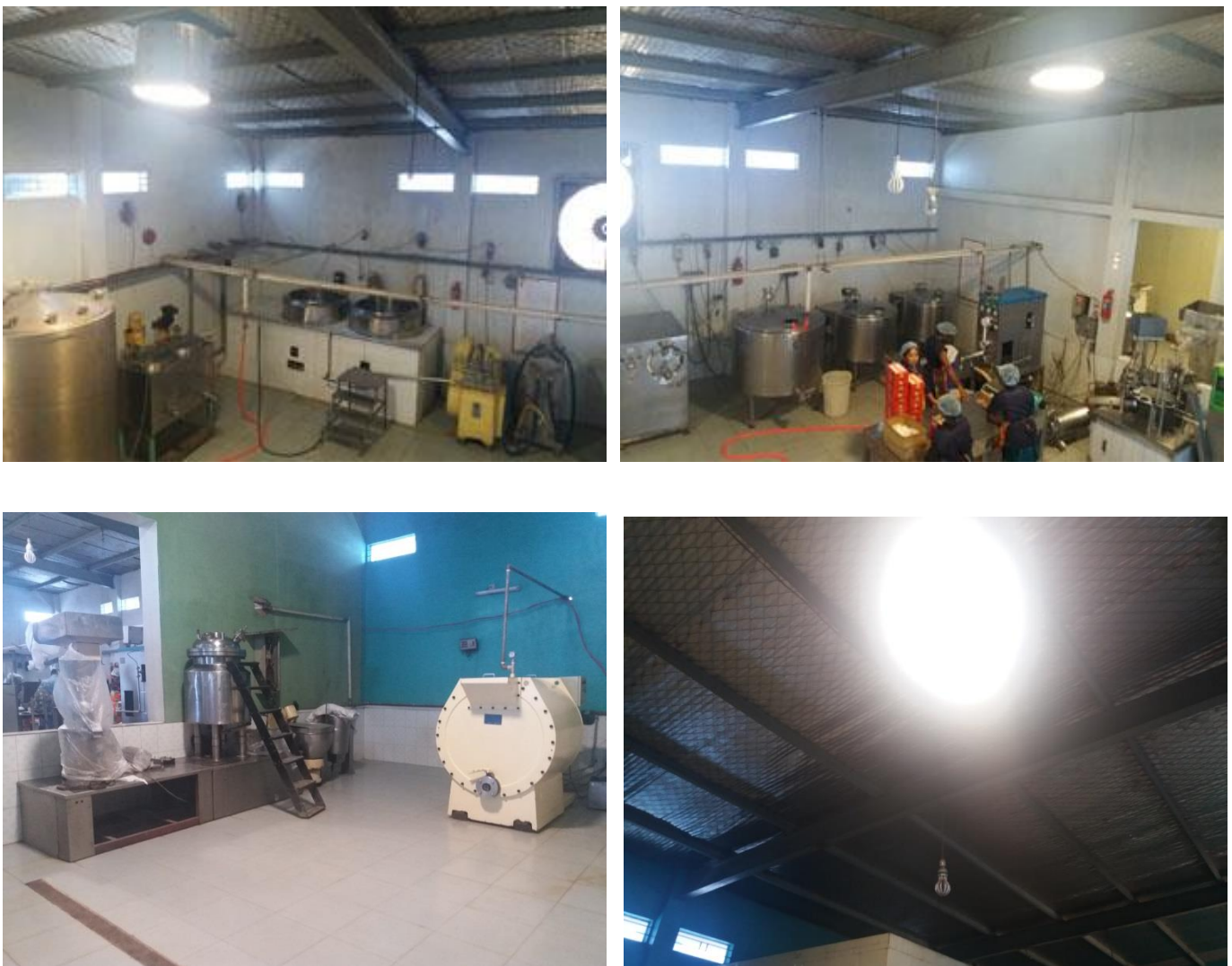
Fig 2: Solar pipe lights installed within the factory.
